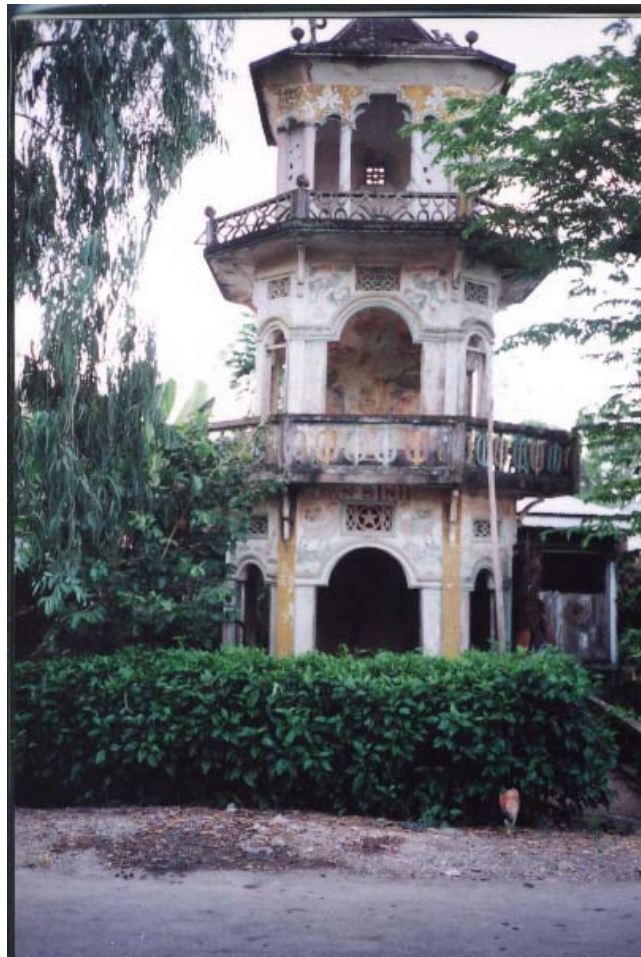
Figure2: A lecture hall turning into ruins
