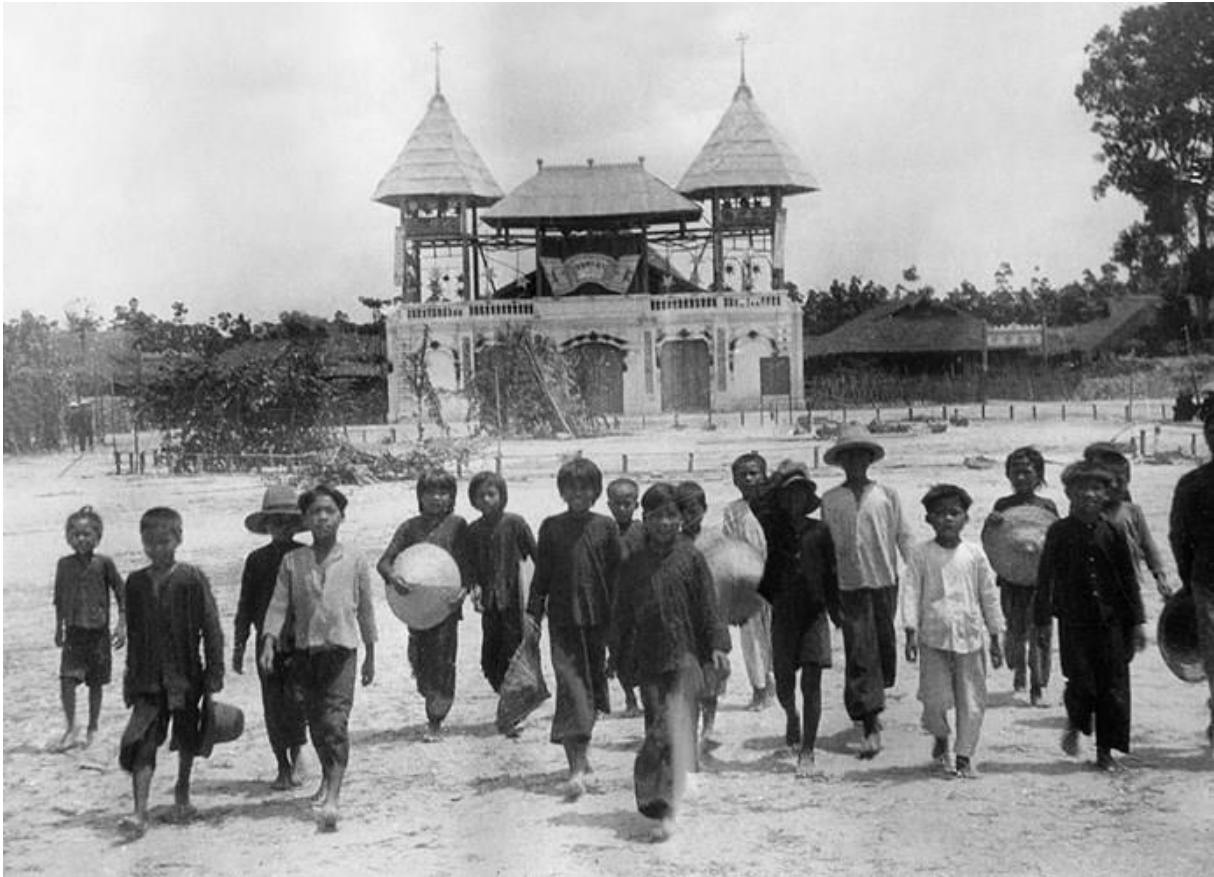
The Cao Dai Religion’s Holy See during construction in 1930, photo by Walter Bosshard
