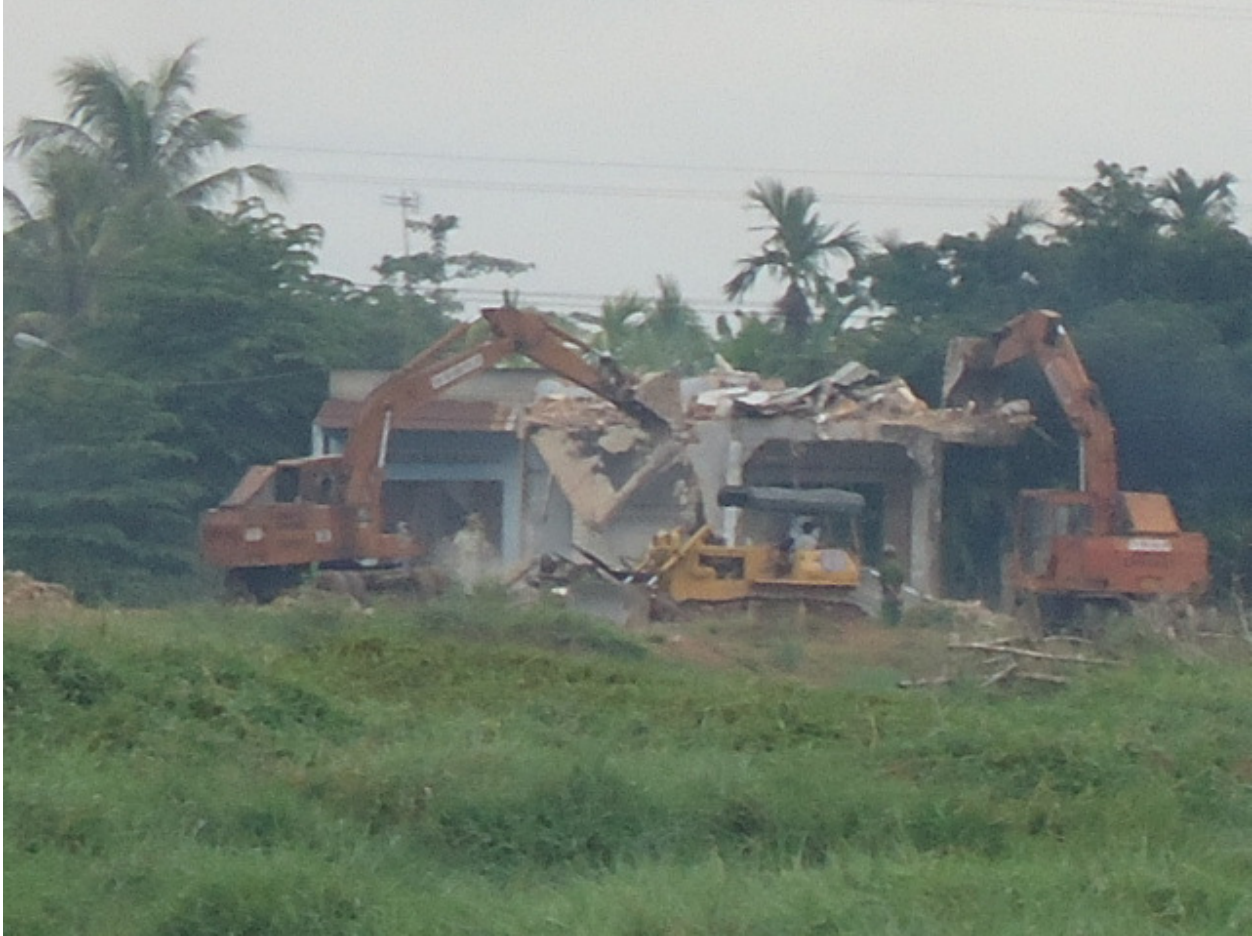
Photo 7: Demolition a parishioner house in June 2013
