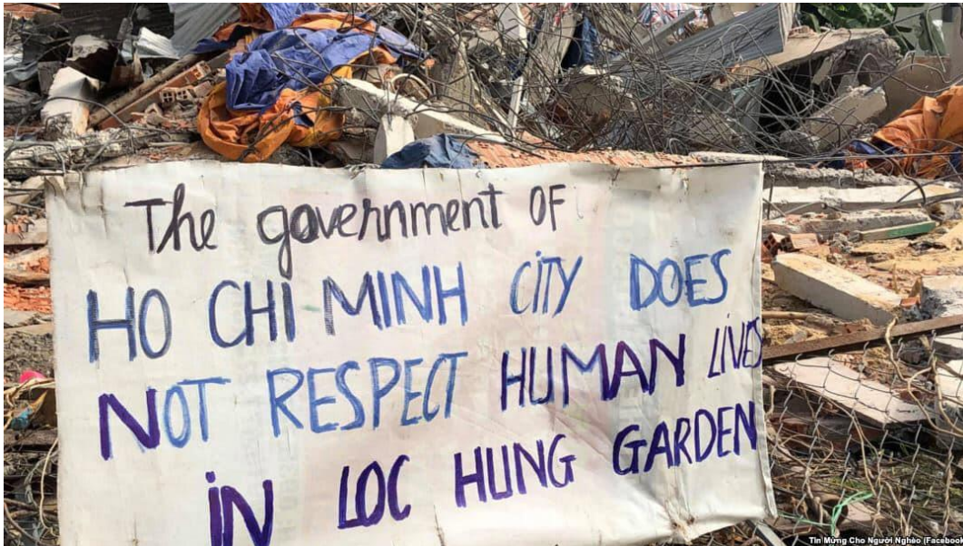
Loc Hung Vegetable Garden after demolition (photo from Facebook)
