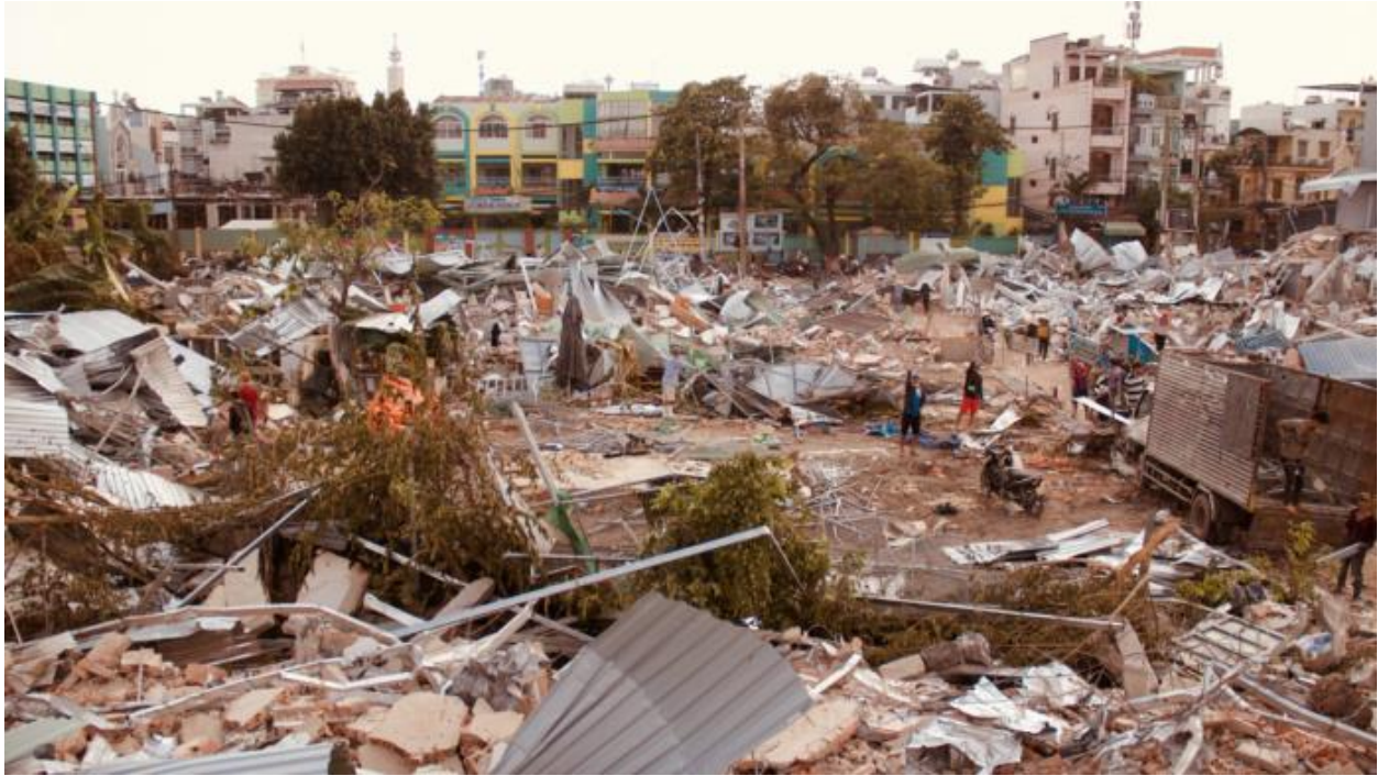
Loc Hung Vegetables Garden after demolition (photo of Nguyen Tri Dung)
